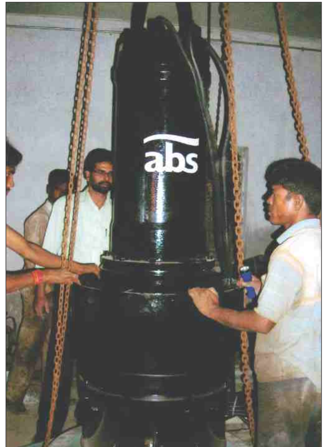
Installation at KMC
